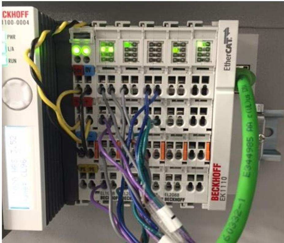
If this does not resolve the fault confirm the address settings on each bank of I/O modules using the address charts below. Each bank of modules will have (1) EK1101 module at the beginning with (3) address dials ( see image below).
