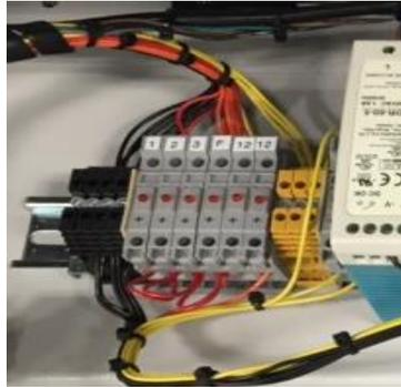
If the voltage here is also below the required 5.3 VDC measure the voltage at the 5V supply located on the left (see image below). The output voltage on the supply must be at its max which is 6.18VDC. If the voltage is below this, use the potentiometer to turn it all the way up. If the supply cannot be turned up to 6.1VDC it must be replaced.
