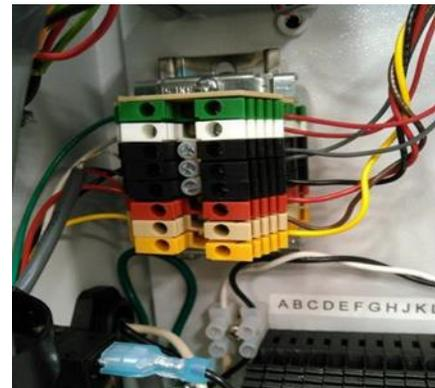
Trim length of each wire for pumps and strip 9mm off of wire and fully insert into terminal block.
