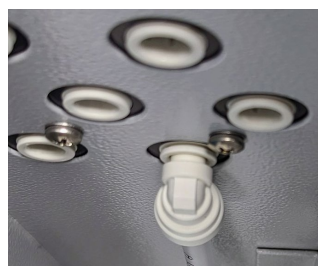
Image 14: Example of fitting not fully seated. Image 15: Example of fitting fully seated.
